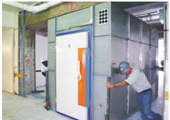
Installation of an exposure unit (reverberation chamber)
